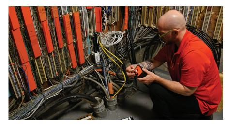
The "meat" of the on-site effort is the Verification Phase of an IVaaS solution. This phase uncovers the inventories of spaces and pathways, including thorough documentation of those inventories—including actions such as cable-label placement, entry-point and conduit mapping, and backbone cable tracing.
