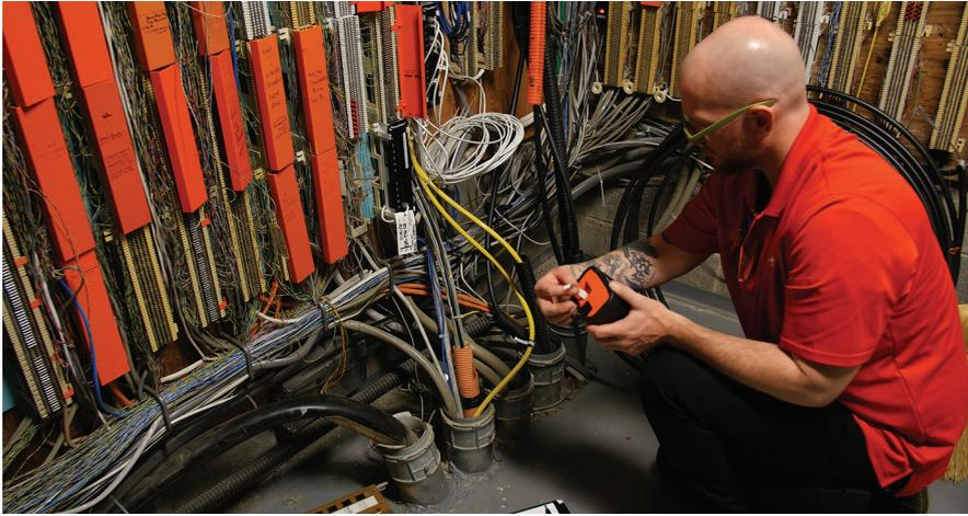
The “meat” of the on-site effort is the Verification Phase of an IVaaS solution. This phase uncovers the inventories of spaces and pathways, including thorough documentation of those inventories—including actions such as cable-label placement, entry-point and conduit mapping, and backbone cable tracing.
